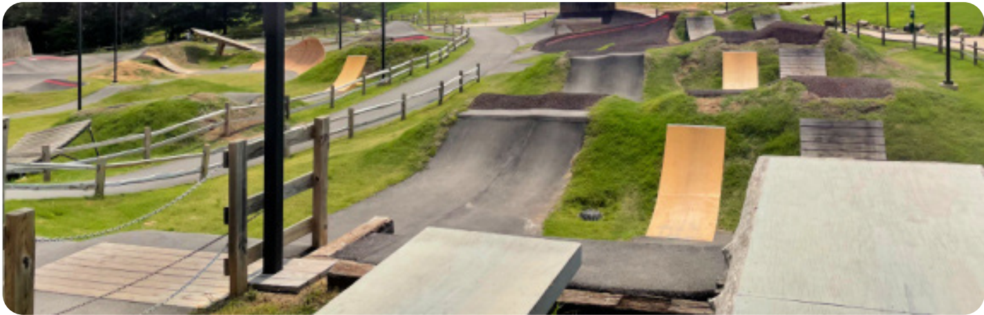
Alignment to accomodate site topography to provide correct grade and subsequent speed of user
